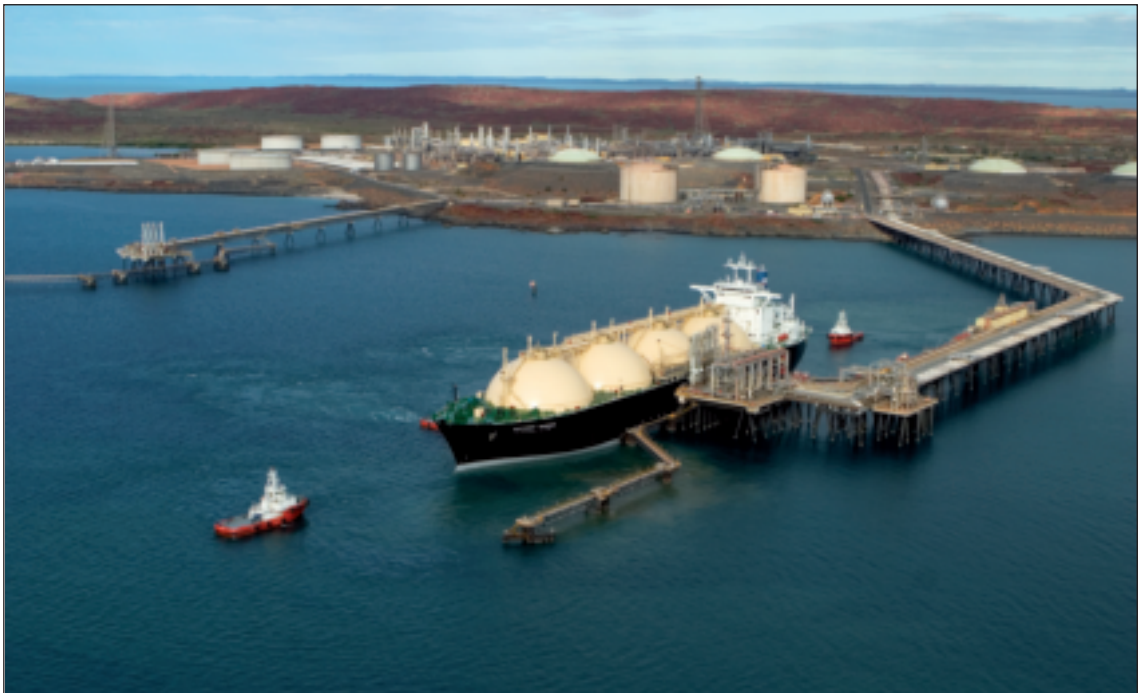
Australia is becoming increasingly important as an LNG supplier – the onshore processing plant at Karratha serving the NWS project.
