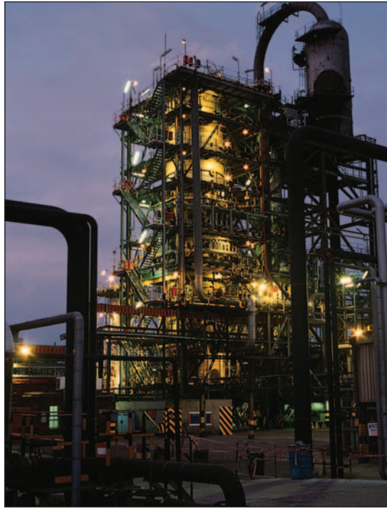
Not many people realise that the gas conversion market is now a similar size to the global LNG trade. Sasol's slurry phase technology will be used in two new GTL plants being developed in Qatar and Nigeria.
