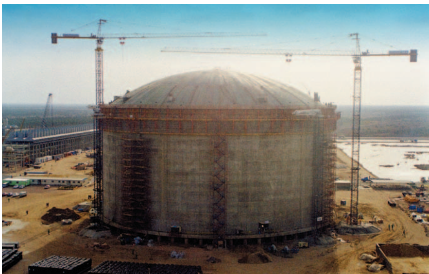
LNG tank under construction in Alexandria, Egypt
