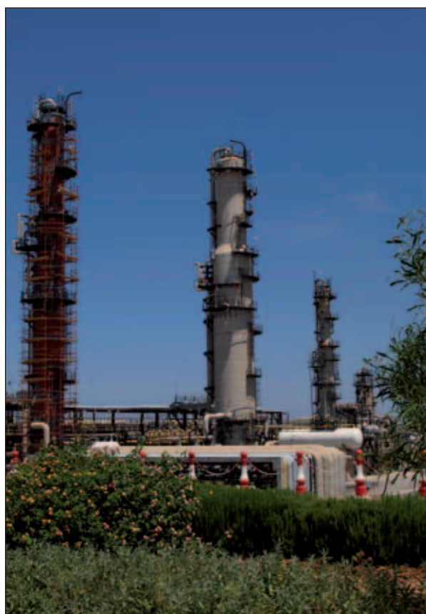
One of Sonatrach's LNG plants located in Arzew, Algeria.
