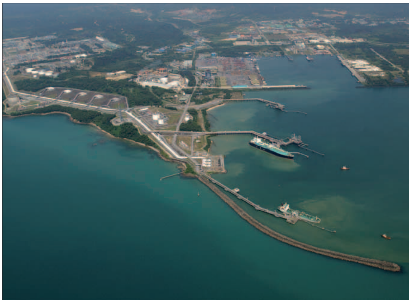
Malaysia is one of the world's largest LNG exporters. The Malaysia LNG plant in Bintulu, which first started production in 1983, has been steadily expanded.
