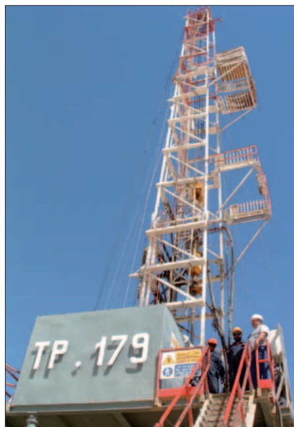
A drilling rig in the south of Algeria.
