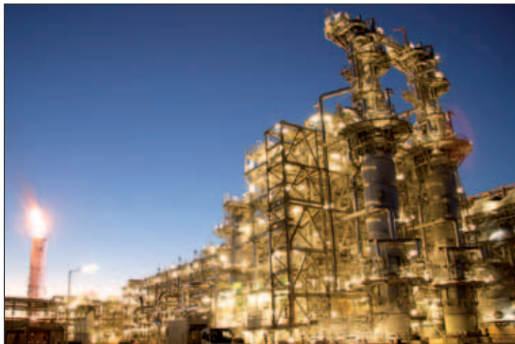
The only new liquefaction capacity to come on stream in 2008 was the fifth train at Australia's North West Shelf plant.
