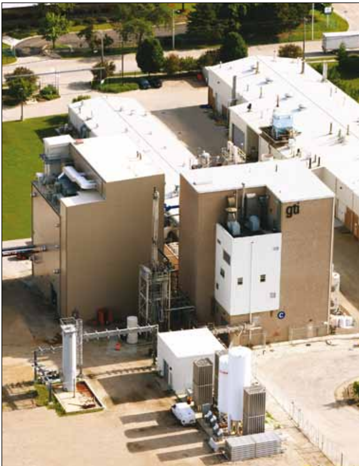
GTI has been involved in gasification R&D for more than 60 years.
