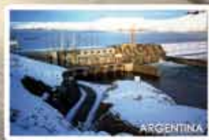
HYDROELECTRIC PICHI PICÚN LEUFÚ ARGENTINA
