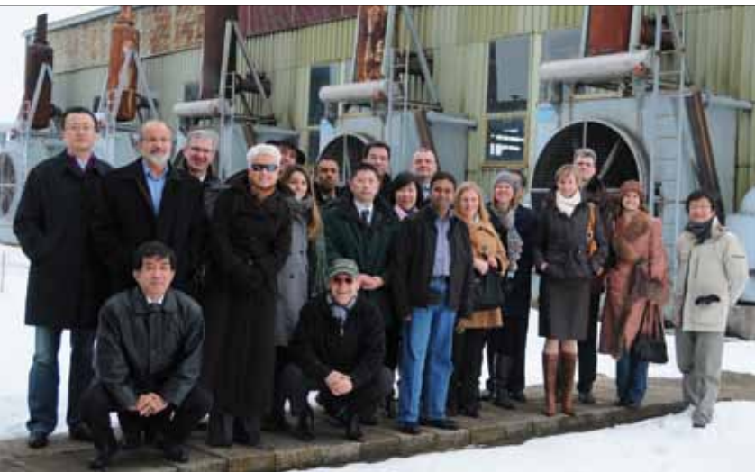
PGC A delegates during their technical visit to the Batajnica compressor station.
