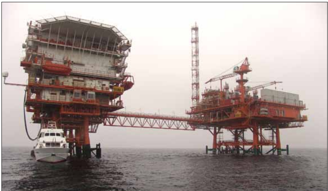
The A and K platforms of the offshore Ivana gas field.
