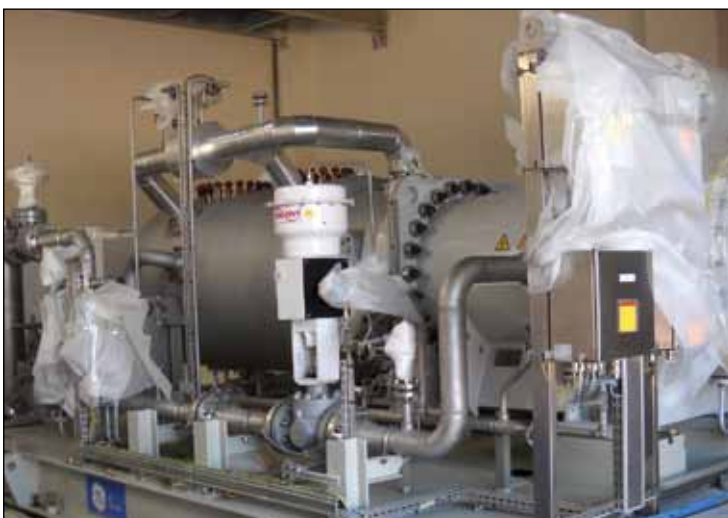
Getting ready to commission an encapsulated compressor at a storage facility.
