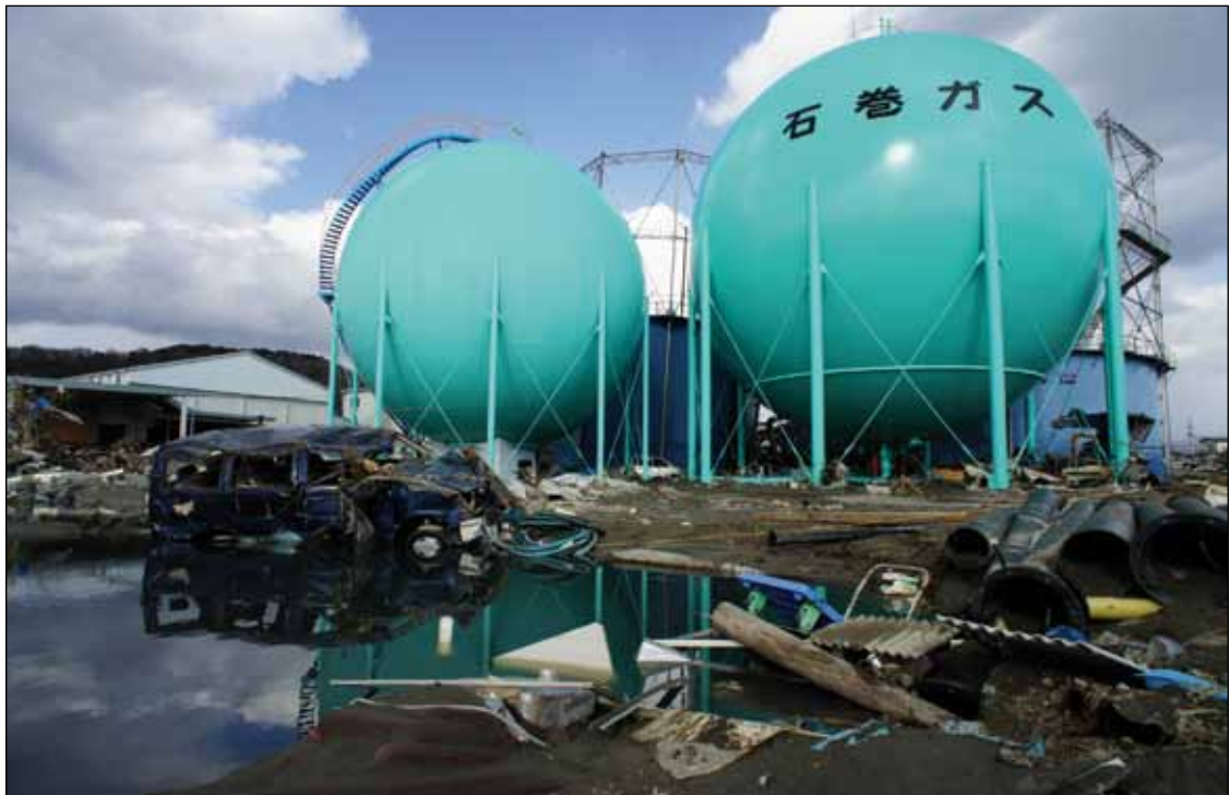
The heavily damaged Ishinomaki gas works in eastern Japan's Miyagi Prefecture after the March tsunami.
