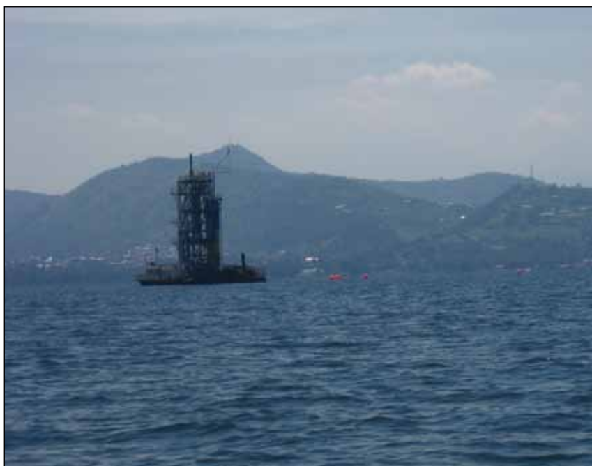
This gas extraction and processing barge for a proof of concept project has been operational since 2008.
