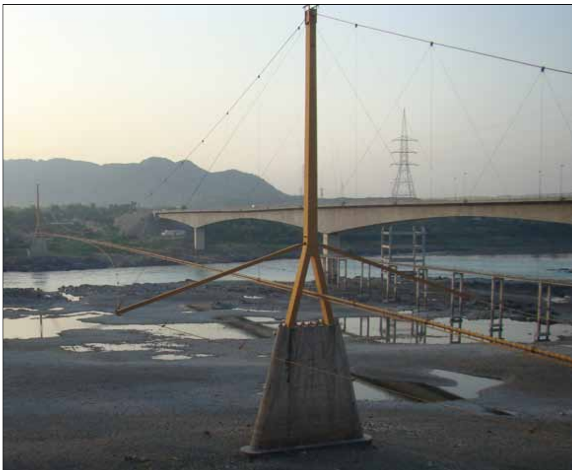
The two main Pakistani gas transmission and distribution companies are Sui Southern (SSGC) and Sui Northern (SNGP). This SNGP transmission pipeline crossing the River Indus by suspension bridge at Khairabad supplies gas to the province of Khyber Pakhtunkhwa in the north of Pakistan.
