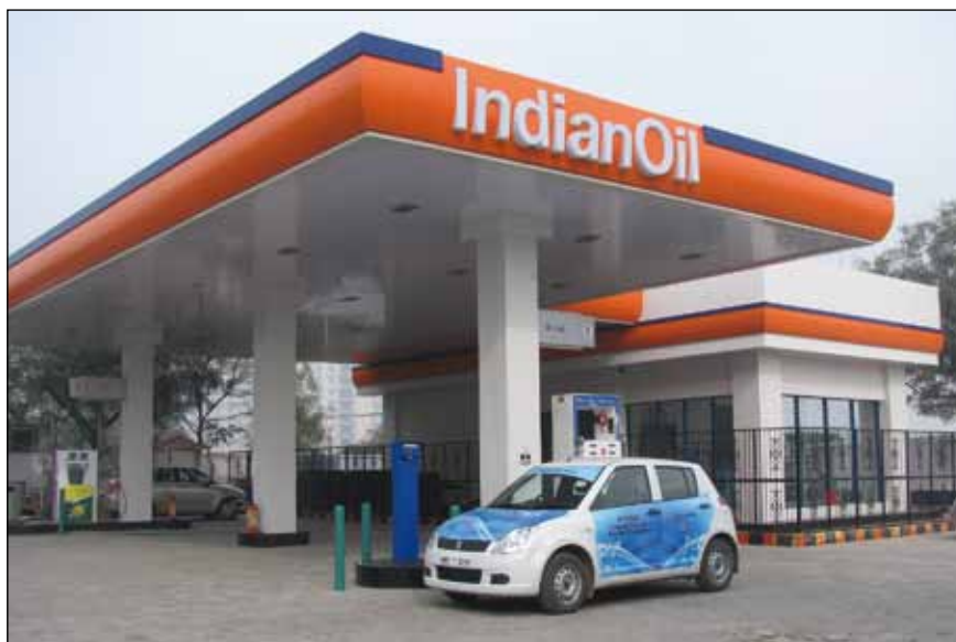
CNG Dispensing Station of IndianOil.
