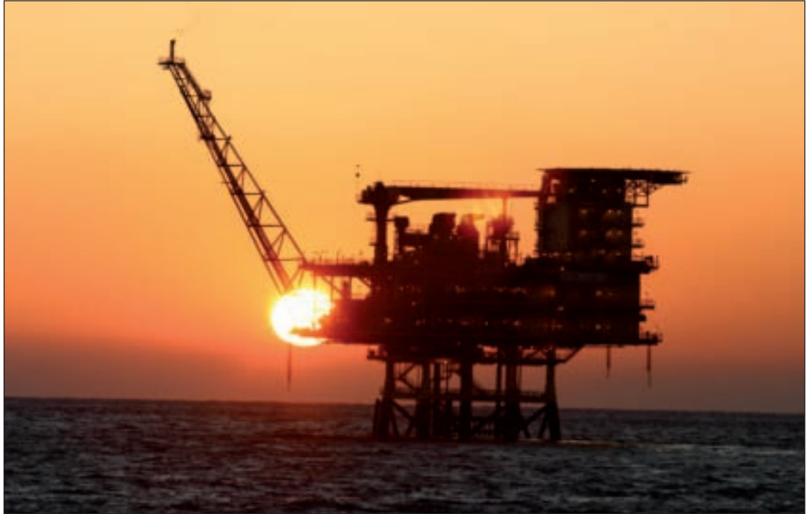
The Donghae-1 gas field is located in Ulleung Basin offshore Ulsan.
