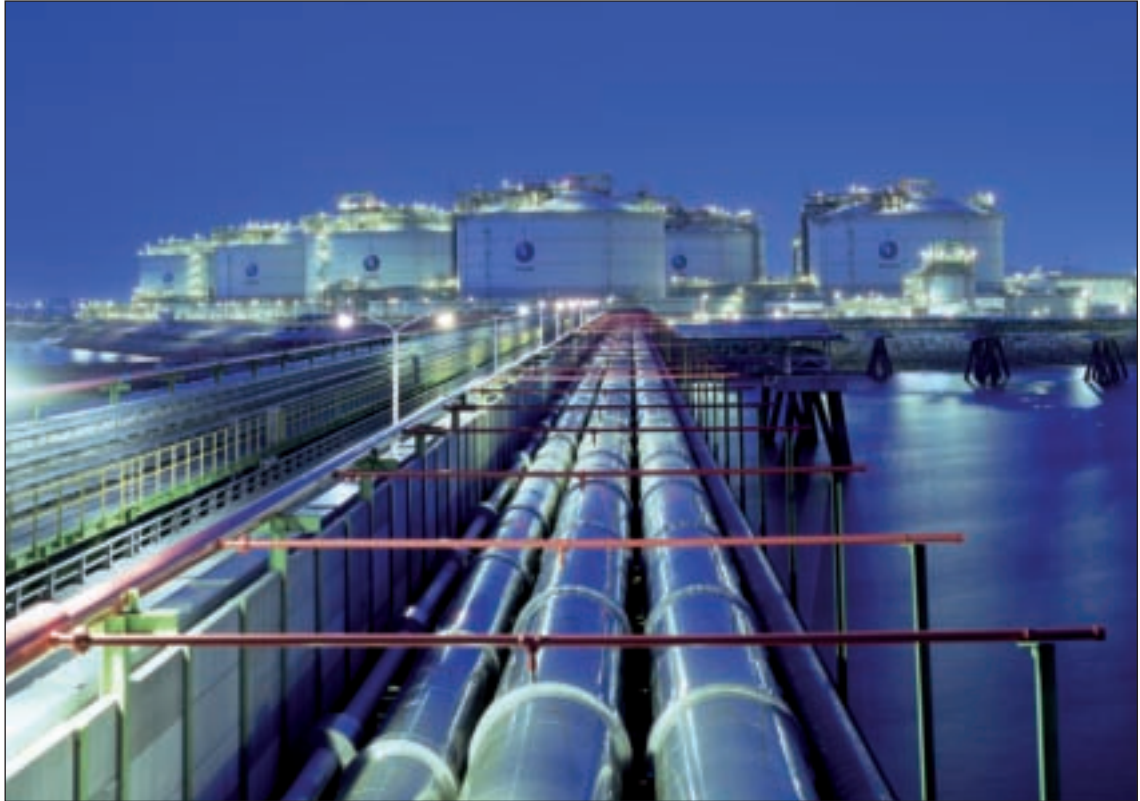
KOGAS operates one of the biggest LNG receiving terminals in the world at Incheon. It entered service in 1996.
