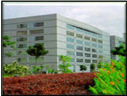
Fuel for Gas District Cooling
