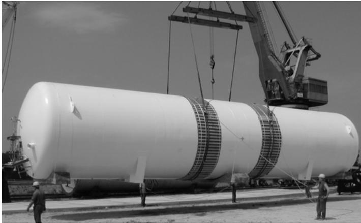
Fig.1. Vacuum insulated tank 403 m<sup>3</sup>
