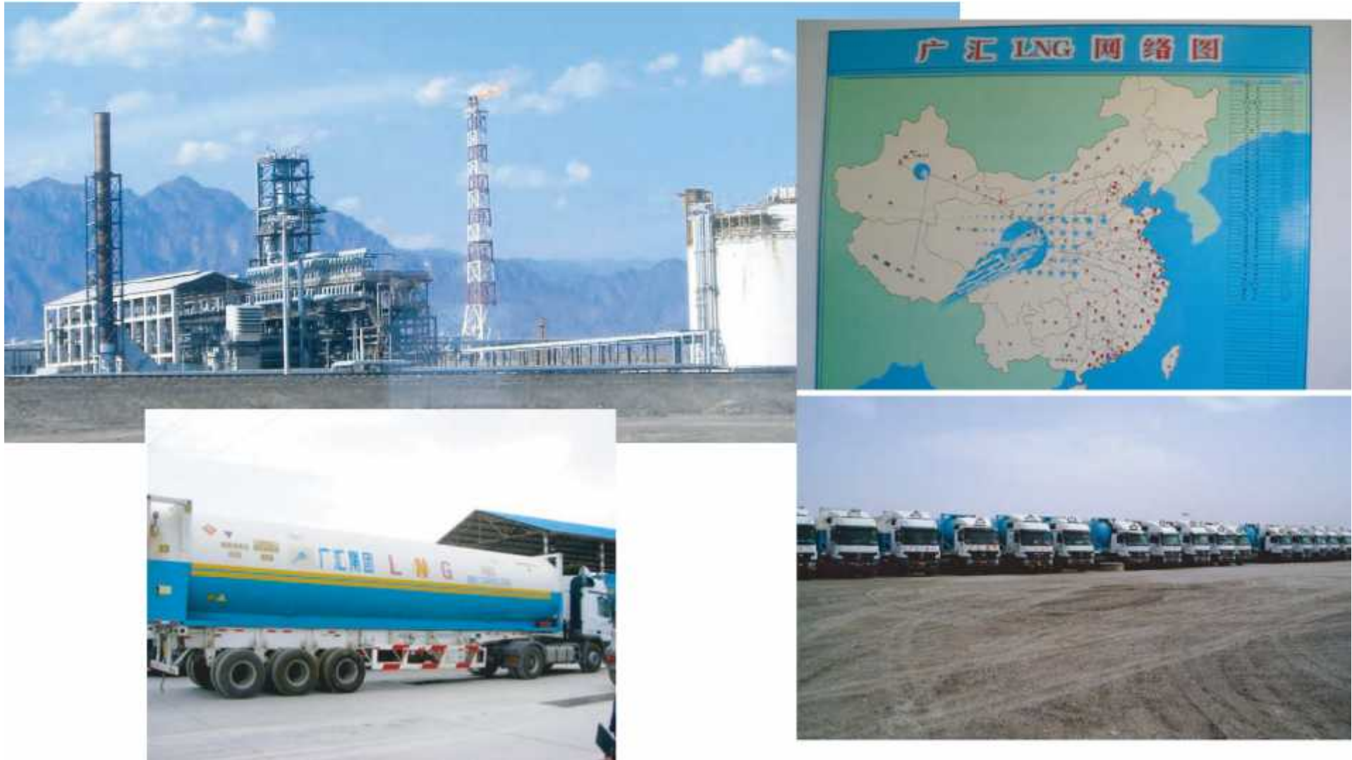
Small-scale LNG plant in Xinjiang by Guanghui LNG is supplied with industrial users in affluent coastal provinces by tank lorry. (pictures) JOGMEC
