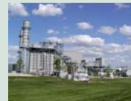
The Riverside Energy Center is a 600 MW combined cycle natural gas-fired electric generating facility located in Beloit, Wisconsin. Cost: $393 million Built: 2004 Area: 3 acres
