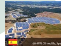
The Olmedilla Photovoltaic Park is a large photovoltaic (solar) power plant in Olmedilla de Alarcón, Spain with 60 MW. Cost: $530 million Built: 2008 Area: 700 acres
