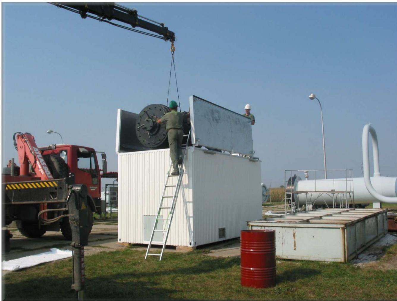
Inserting to the work space
